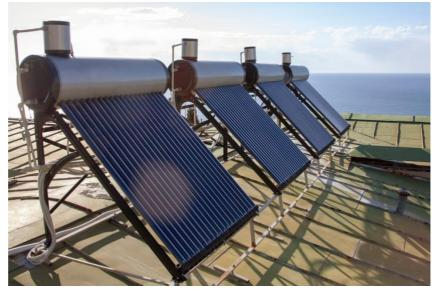
low sunlight intensity, occurring on winter days in cloudy or foggy regions such as Austria, it is necessary to complement the solar thermal system with supplementary heat generators such as boilers or heat pumps to ensure a continuous supply of heat.
